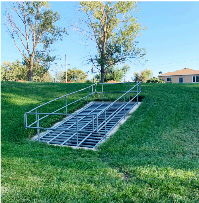
Large stormwater culvert grate at Citizen's Park
